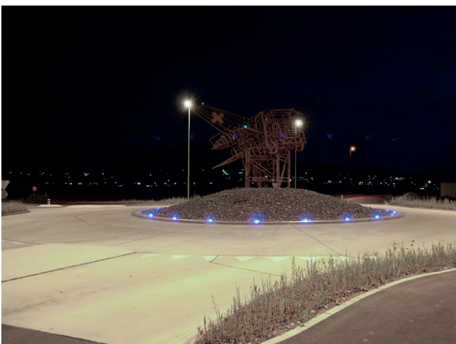
CircLED roundabout Bachenbülach
