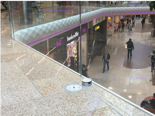
Floor socket outlet Fonto and Masso, shopping centre Plus City
